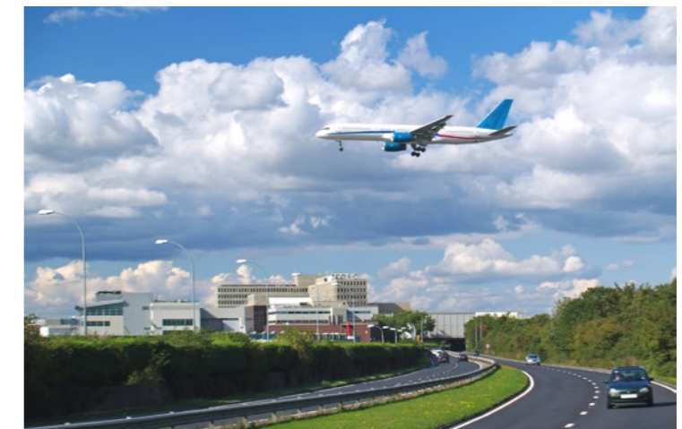
Figure 43. Gatwick Airport. South Terminal and Road Tunnel
